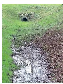
The impact of a drainage system on the surrounding plots also needs to be carefully considered. For example, if an overflow directs heavy rainfall off the plot it could result in flooding in a neighbouring plot.
